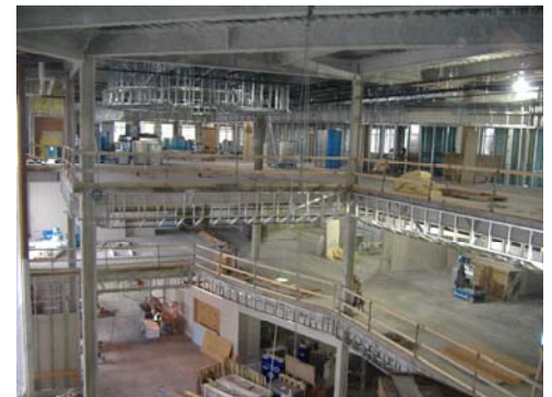
On 3 rd Level looking into Atrium toward Coffee Shop
