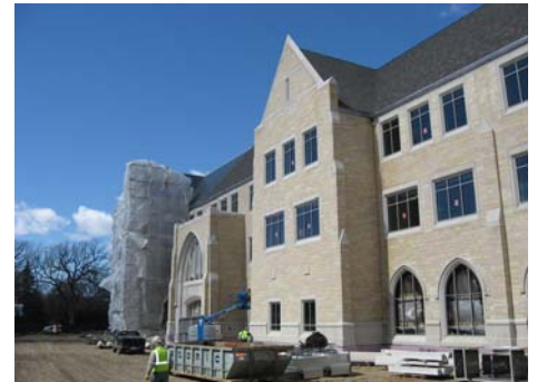
South Exterior & Building Entry
